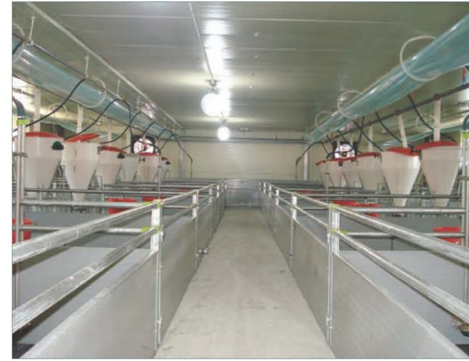
Case of an installation (incubator foundation)
