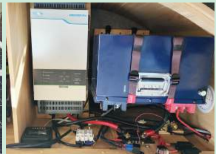
600A Lithium Iron Phosphate battery
