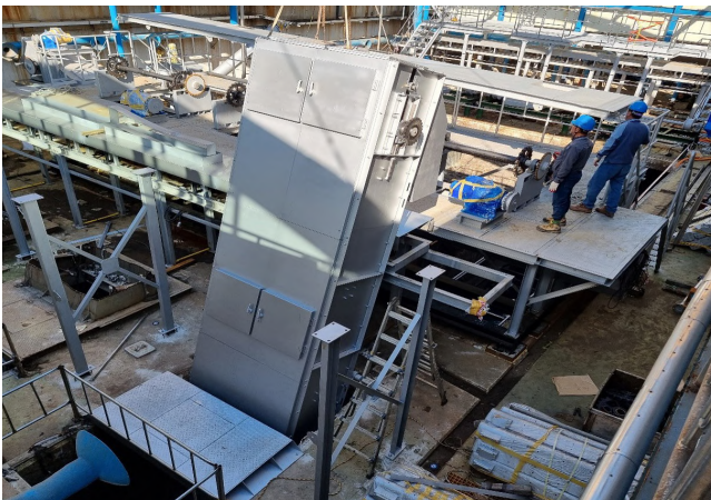
Installation of fine screen at Jeonju Sewage Treatment Plant in Jeonbuk
