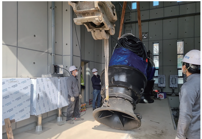
Delivery of column pipes and Mixed flow pumps to Gangseo-gu, Busan
