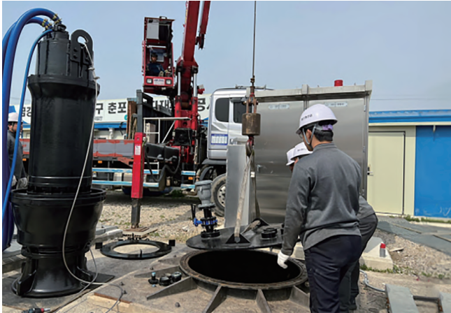
Delivery of Mixed flow pump to Ganri pumping station
