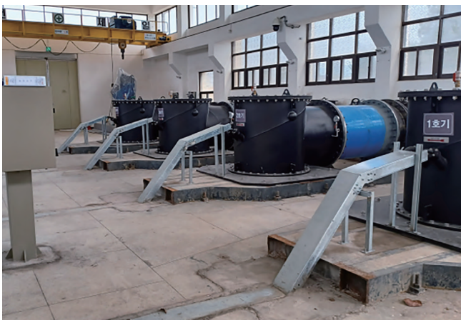
Delivery of Mixed flow pump to Namwon Gwiseok Drainage Plant
