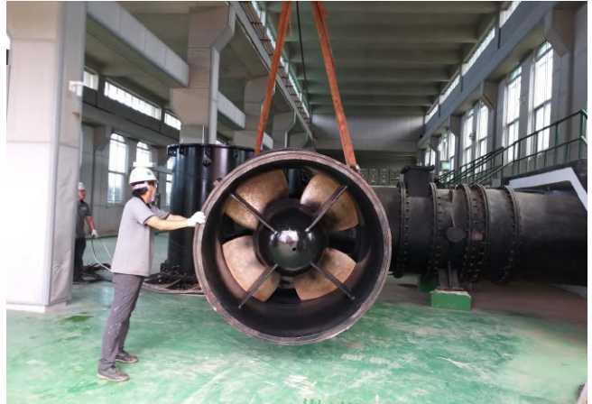
Delivery of Axial flow pump to Jeongeup Gukjeong Pumping & Drainage Station
