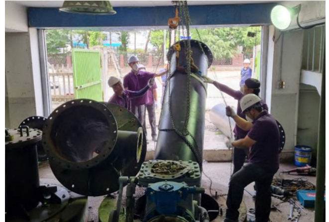
Column installation at relay pump station in Iksan, Jeollabuk
